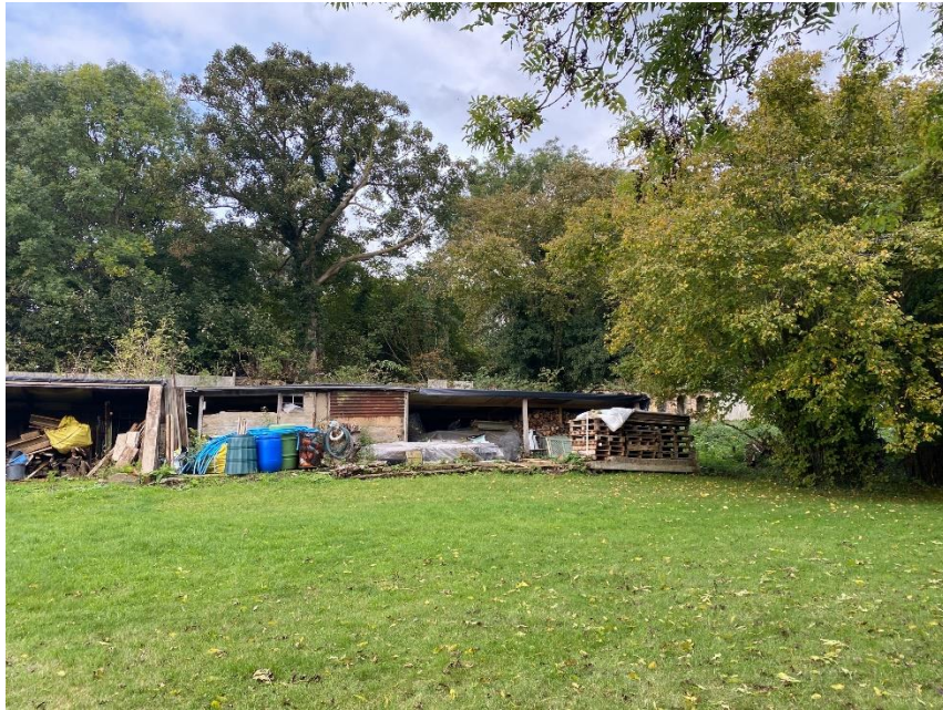
The line of concrete, derelict sheds that will be removed to open up the view of the Arcaded Wall
