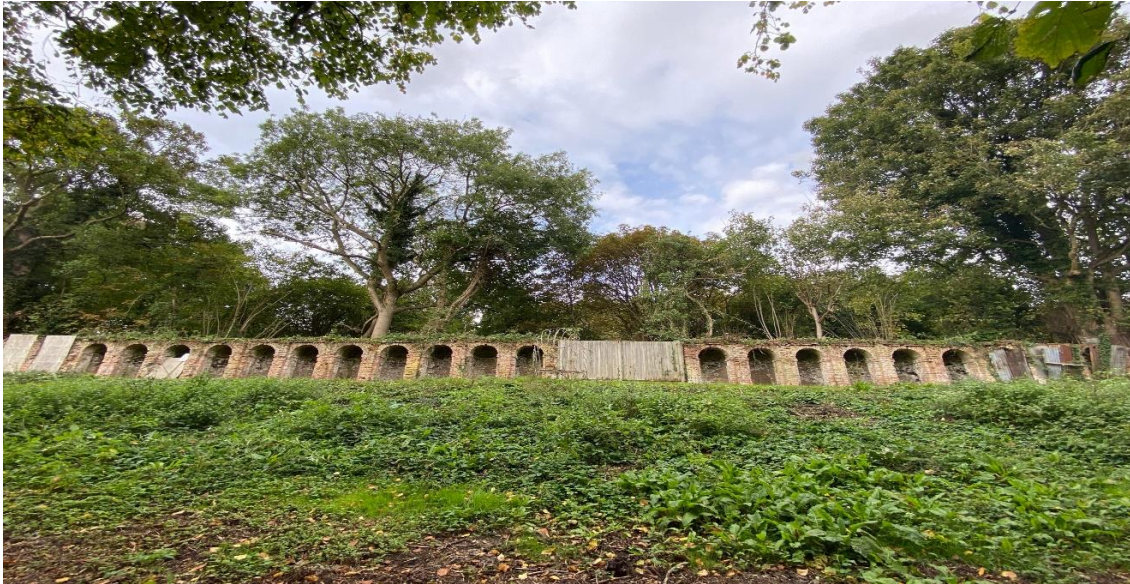
The Arcaded Wall in the Orchard, 2020, after tree removal work was completed
