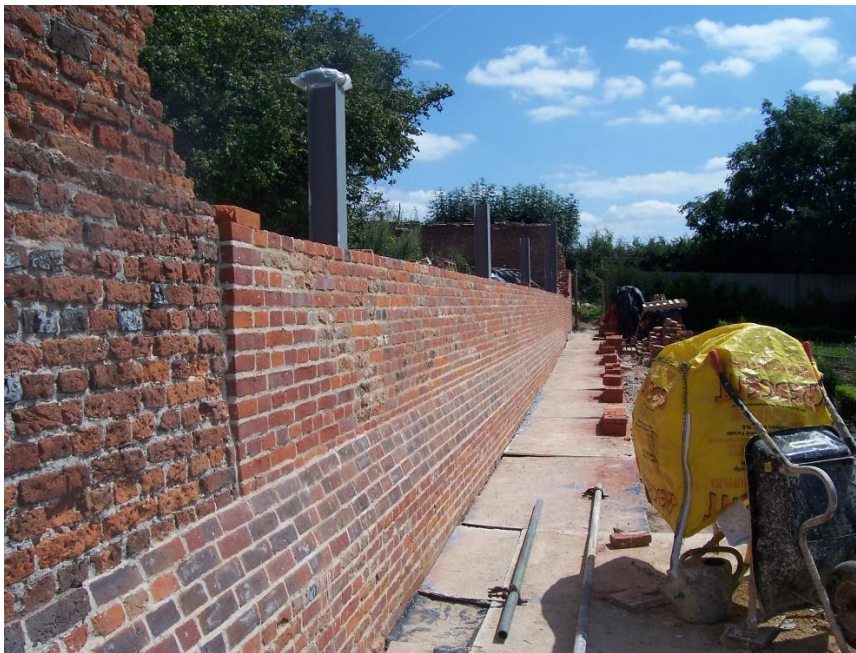
The Eastern Wall under construction
