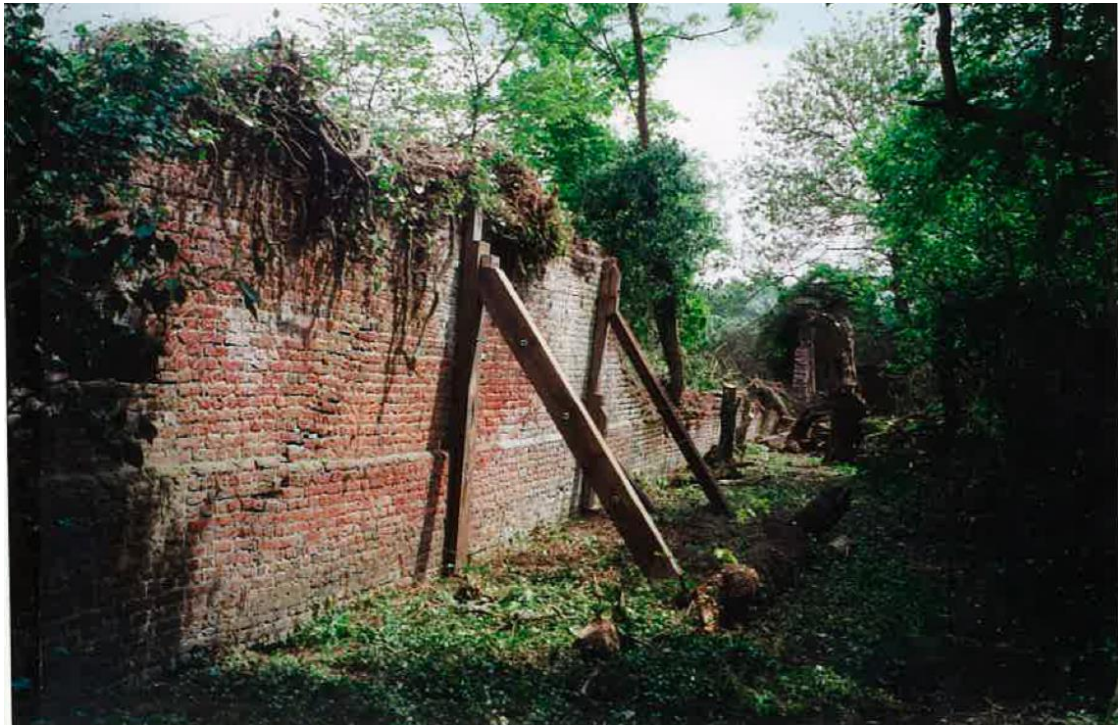
Eastern Orchard Wall in 2004 with temporary supports
