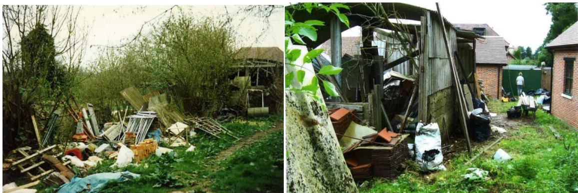
Existing asbestos shed and rubbish pile on planned site of the Proposed Outbuilding, already cleared
