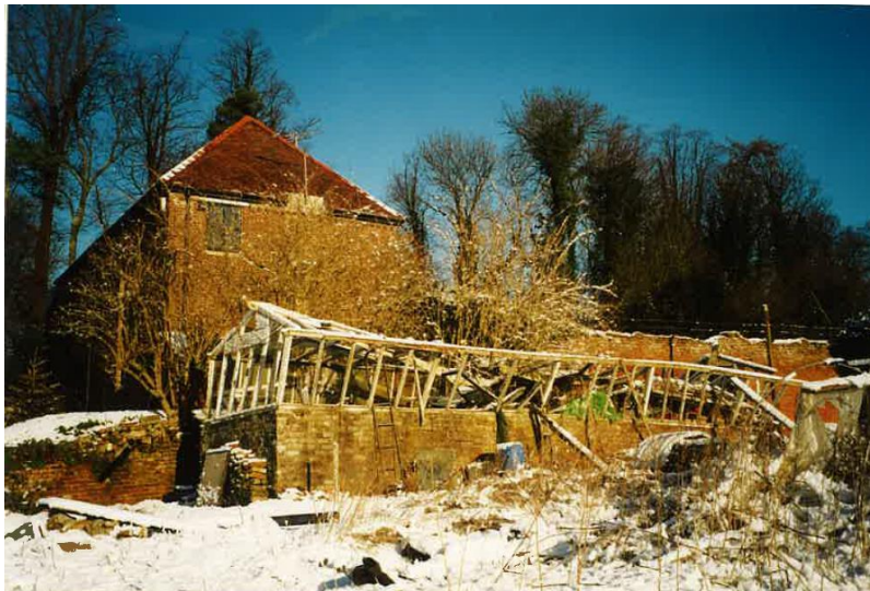
The Glasshouse in the Kitchen Garden in 2002, damaged by flood water escaping from the Orchard
