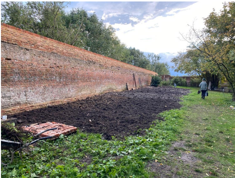
The Southern Boundary Wall in the Orchard, 2020, with trees cleared and minor repairs underway
