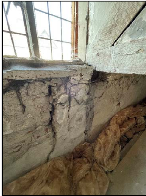
Figure 4 – Cracking at Location of Truss Bearing
