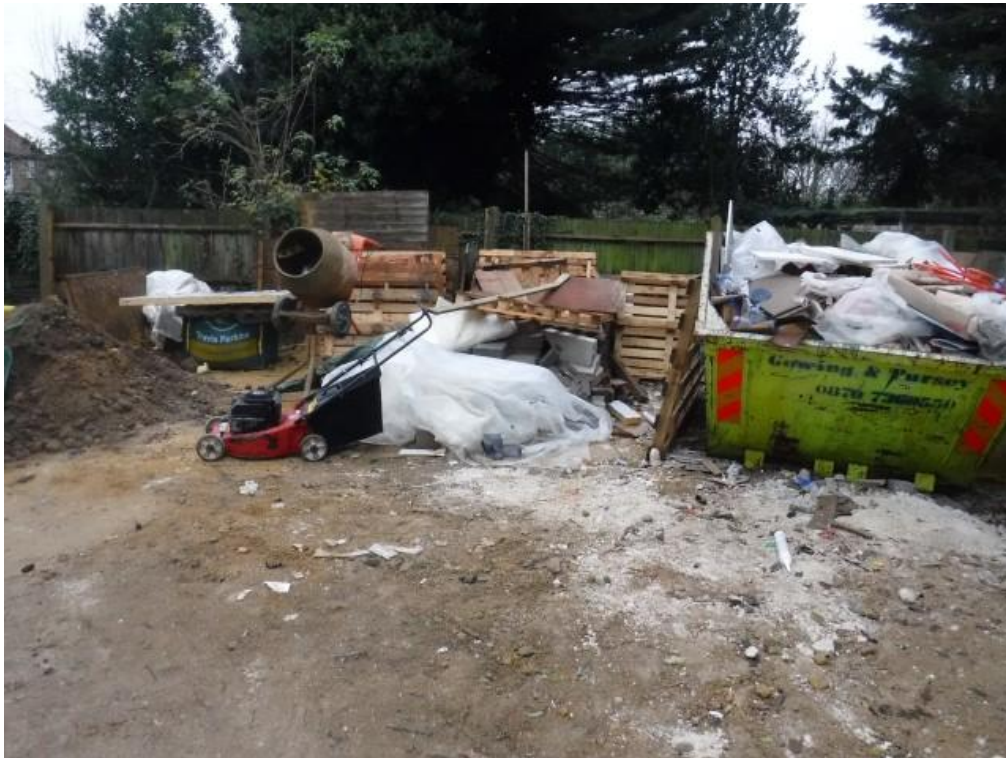
Rear of No. 583 Uxbridge Road
