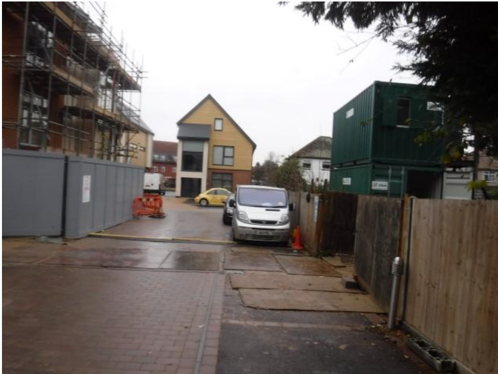
Looking northerly from south of site. No. 583 Uxbridge Road in background (right)
