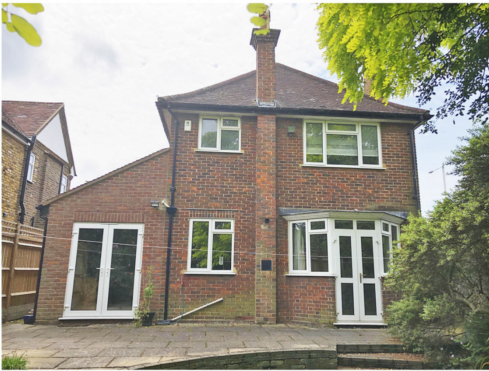
PHOTO 2: VIEW OF EXISTING REAR ELEVATION
