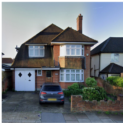
Fig 01 – No. 8 Belmont rd with catslide roof
