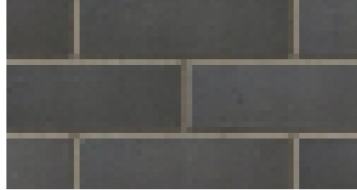
Ibstock Staffordshire Slate Blue Bricks Below DPC
