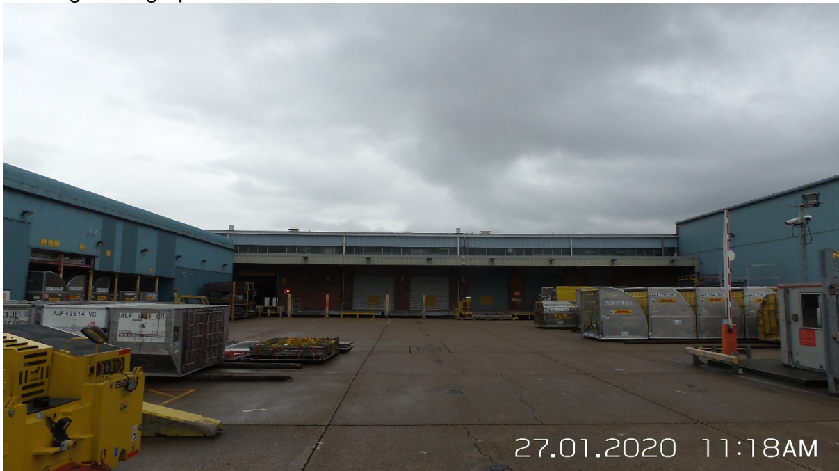
Existing Service Yard Airside View from internal access road
