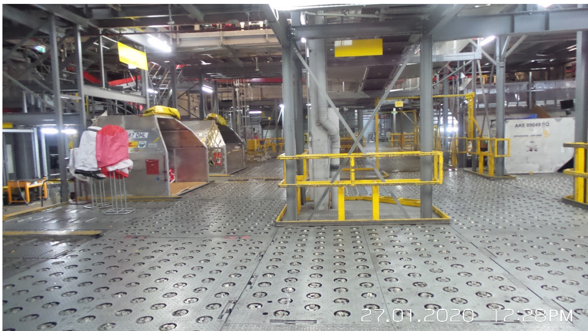
Internal view of Warehouse with roller casters to move ULD's around
