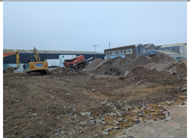
Photo 6: View towards the southeast with floor slab having been removed and the site levelled, and a concrete crusher to the rear with stockpiles of crushed concrete.
