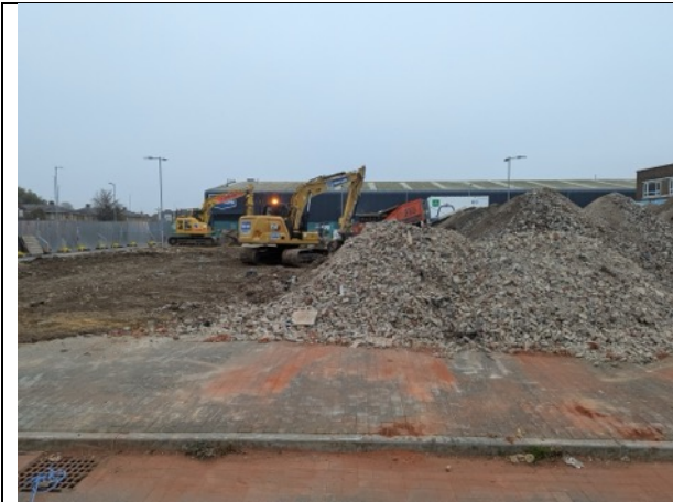
Photo 5: View towards the east with the site levelled and crushed concrete stockpiled in the south of the site.
