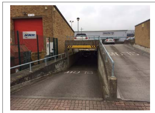
Access ramps for twin-deck car park (CBRE 2018)
