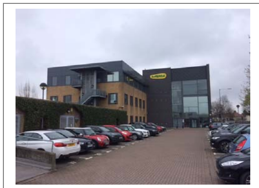
General view of building, car park and plant enclosure/ESS (CBRE 2018)
