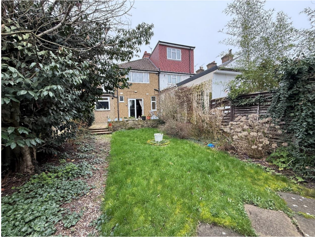
Rear view towards adjoining neighbour No.32
