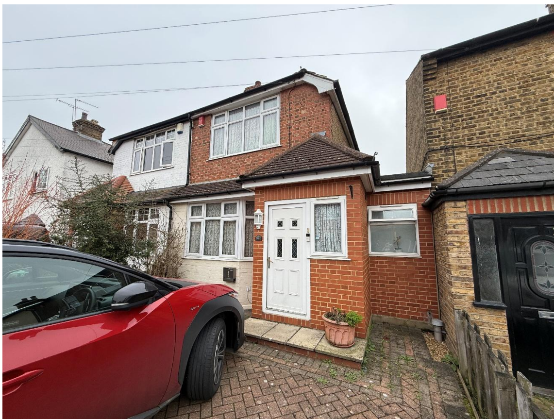
Front view towards adjoining neighbour No.32
