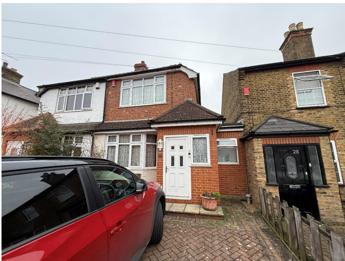
Front view towards neighbour No.28
