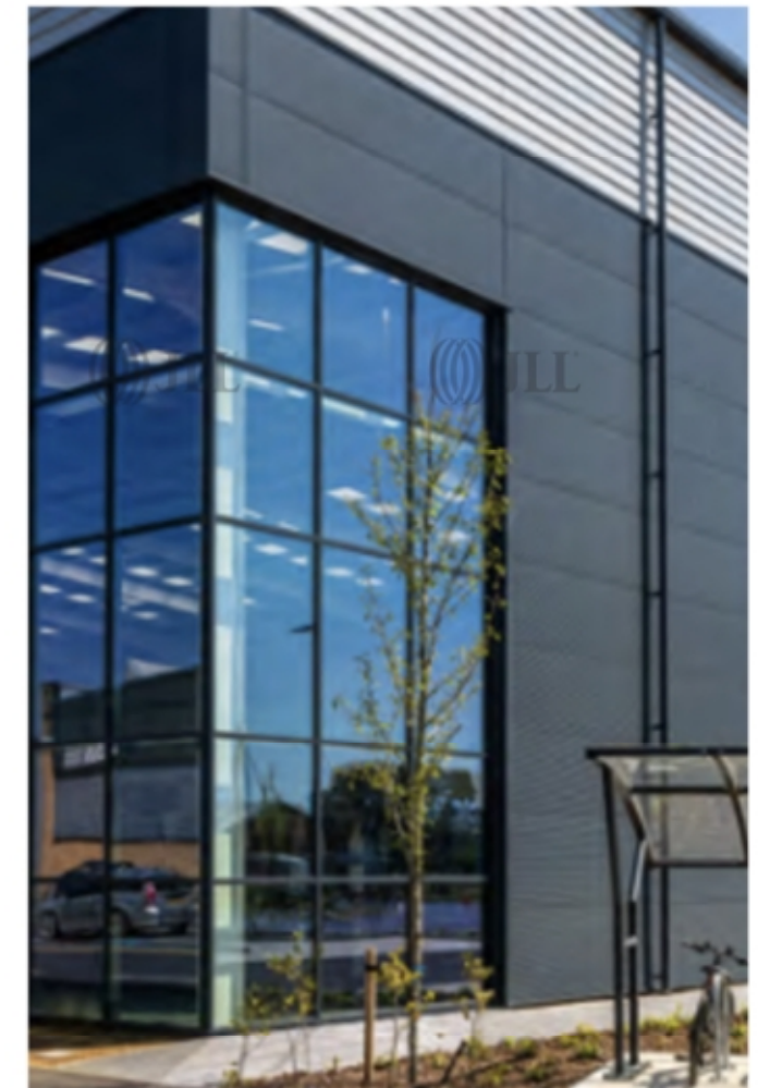
6. Curtain wall glazing
