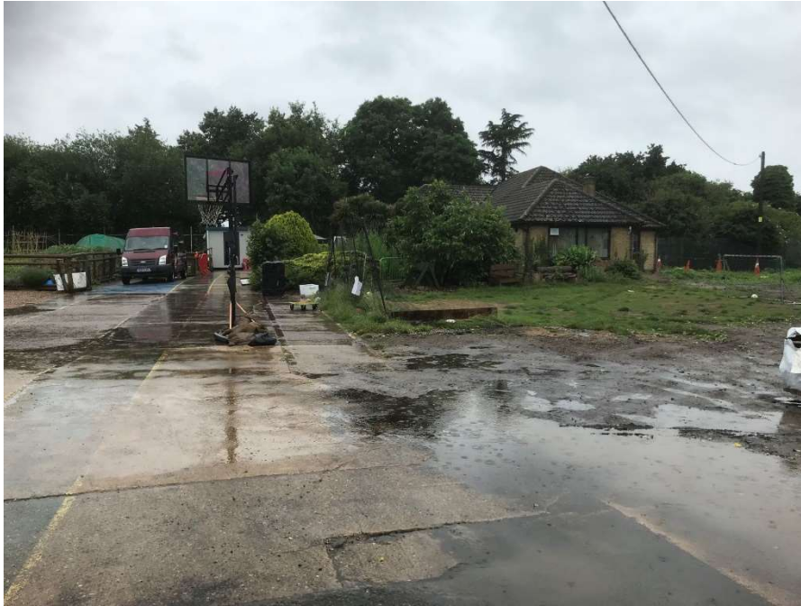
Image 1: Looking west across the Site towards the reception building
