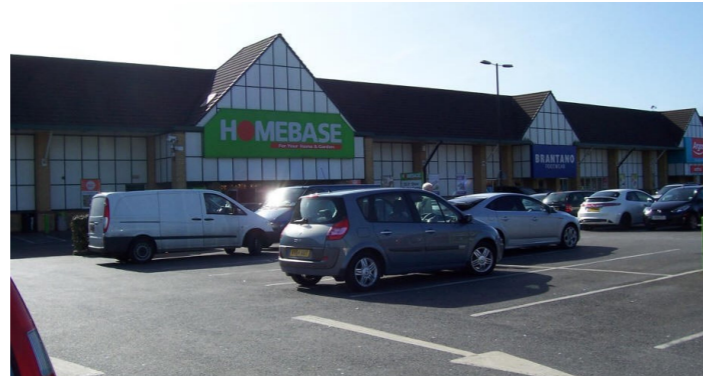
2 | Frontage of the Former Homebase
