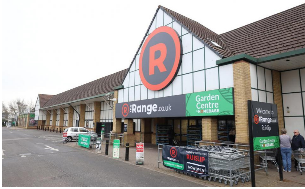
A photo of the existing storefront to Unit 1
