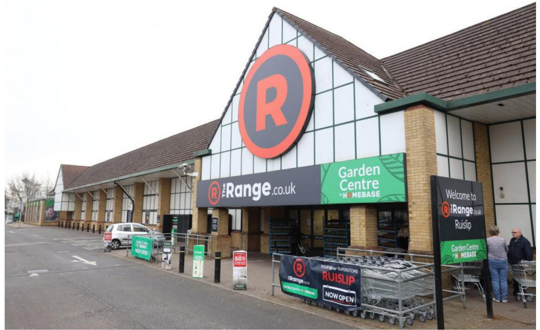
A photo of the existing storefront to Unit 1, Victoria Retail Park
