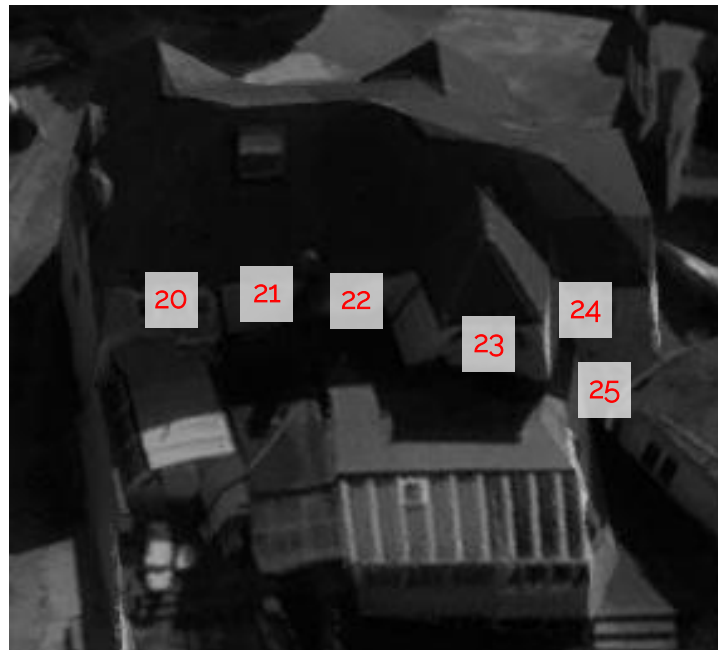
Gateway Court (Rear Elevation)
