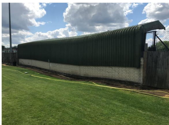
Existing stand showing settlement of ground
