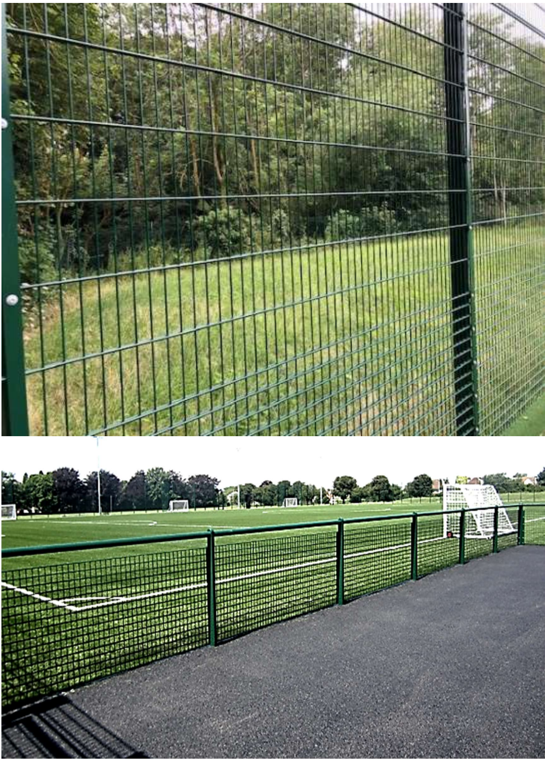
Rigid panel ballstop fencing to perimeter of the pitch
