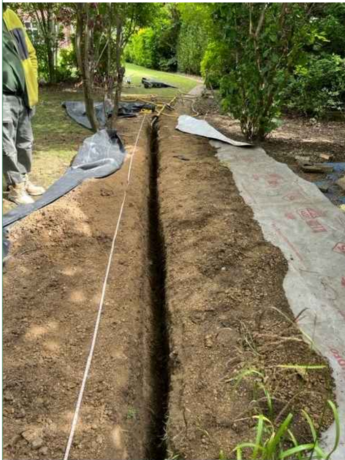
01 - Location of 8m trench excavated by air-spade to a depth of 0.7m, 0.3m beyond footprint of approved garden office.
