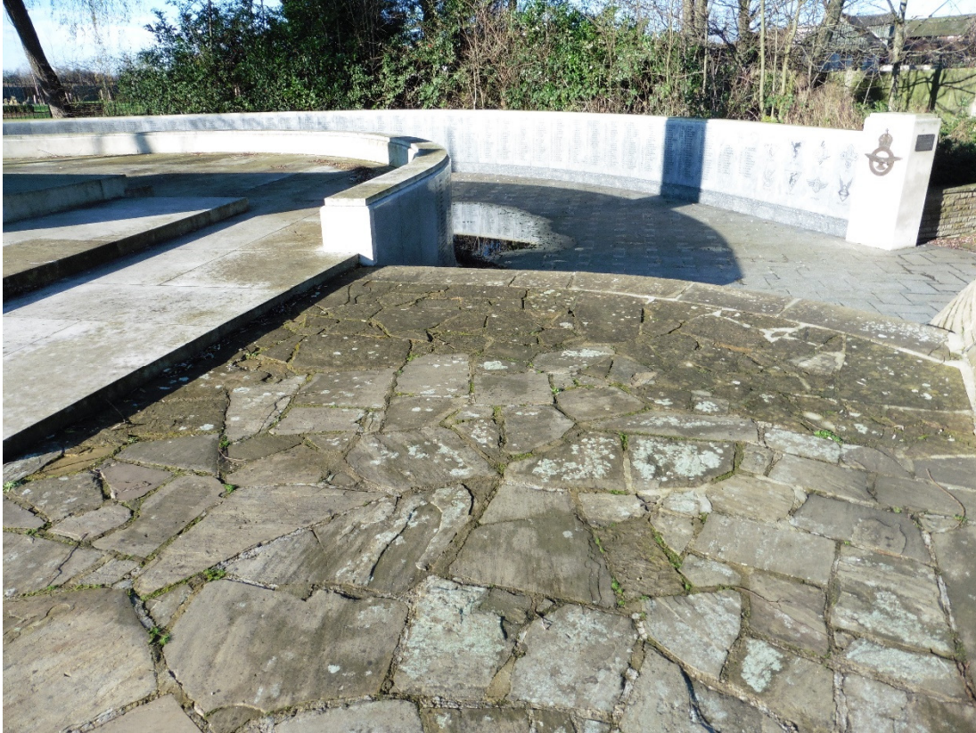
Picture 5. Showing York paving with open joints and with some vegetative growth
