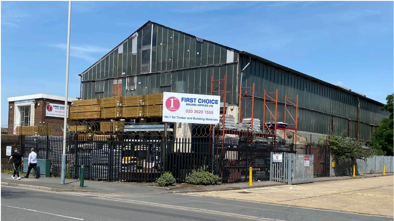
VIEW FROM EAST PUMP LANE
