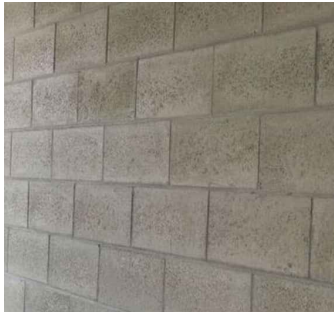
MASONRY PLINTH 140mm FAIR FACED CONCRETE BLOCKWORK
