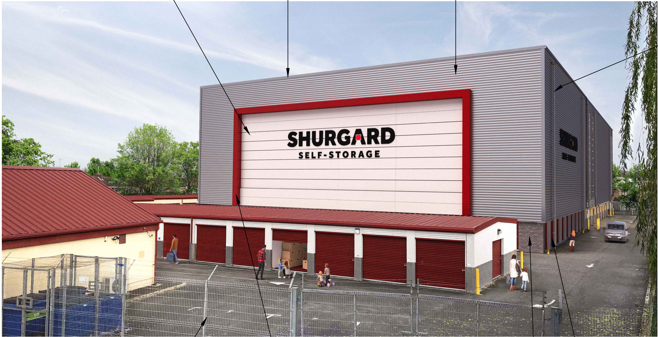
EXTERNAL WALL CLADDING - Contrasting Panel Zone - Horizontal KINGSPAN QUADCORE AWP KS1000 MR MICRORIB RAL 9003 - White
