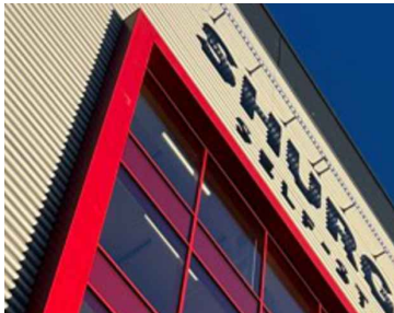
FEATURE ARCH PPC ALUMINIUM FLASHING TRAFFIC RED RAL 3020
