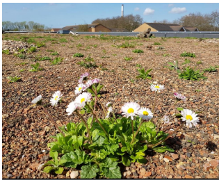
ROOF PANEL (Behind parapet) Brown Bio-Diverse Roof
