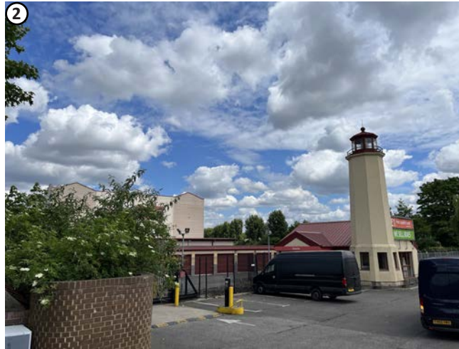
Plate 2 View from north east towards the site from the Uxbridge Road.
