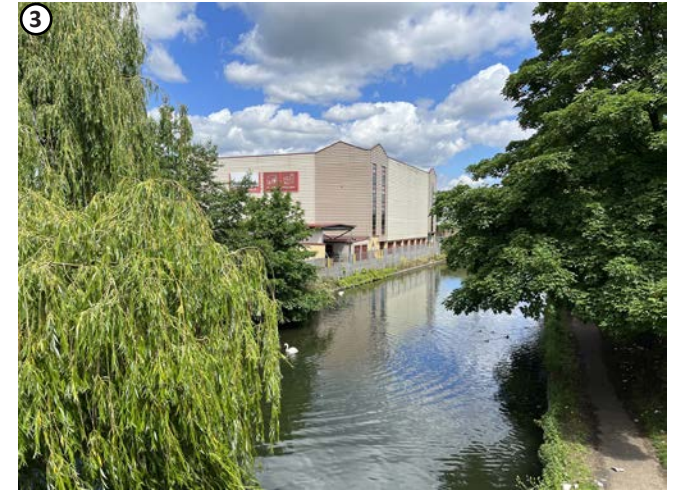
Plate 3 View looking north west towards the site from the bridge on the Uxbridge Road.
