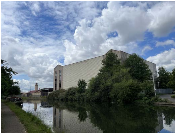
Plate 11 The site as seen from the tow path. The building has a negative impact aesthetically but reinforces the industrial character of the area.
