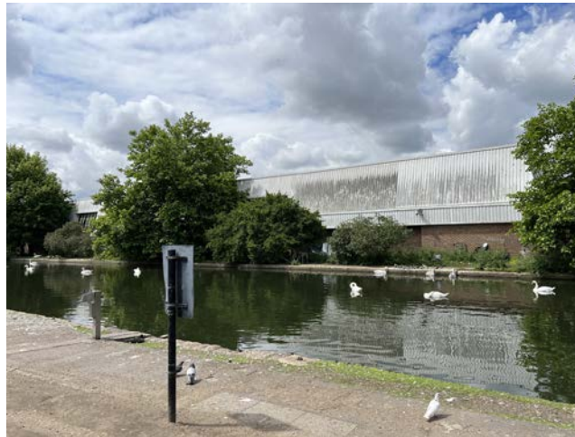
Plate 14. Industrial unit to the south of the conservation area, aesthetically detract but reinforce industrial character.
