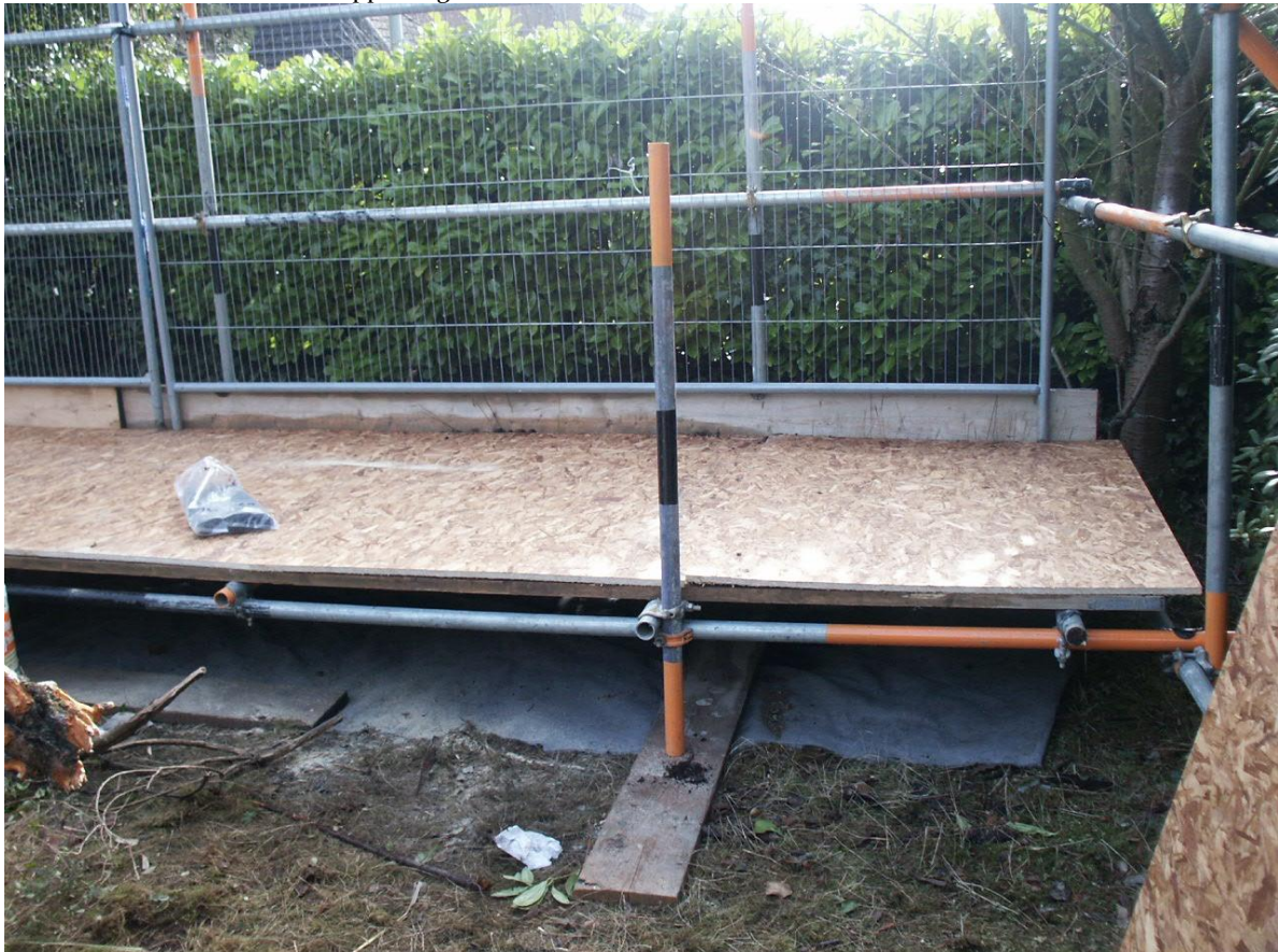
Photo 2 Scaffold framework supporting wooden boards
