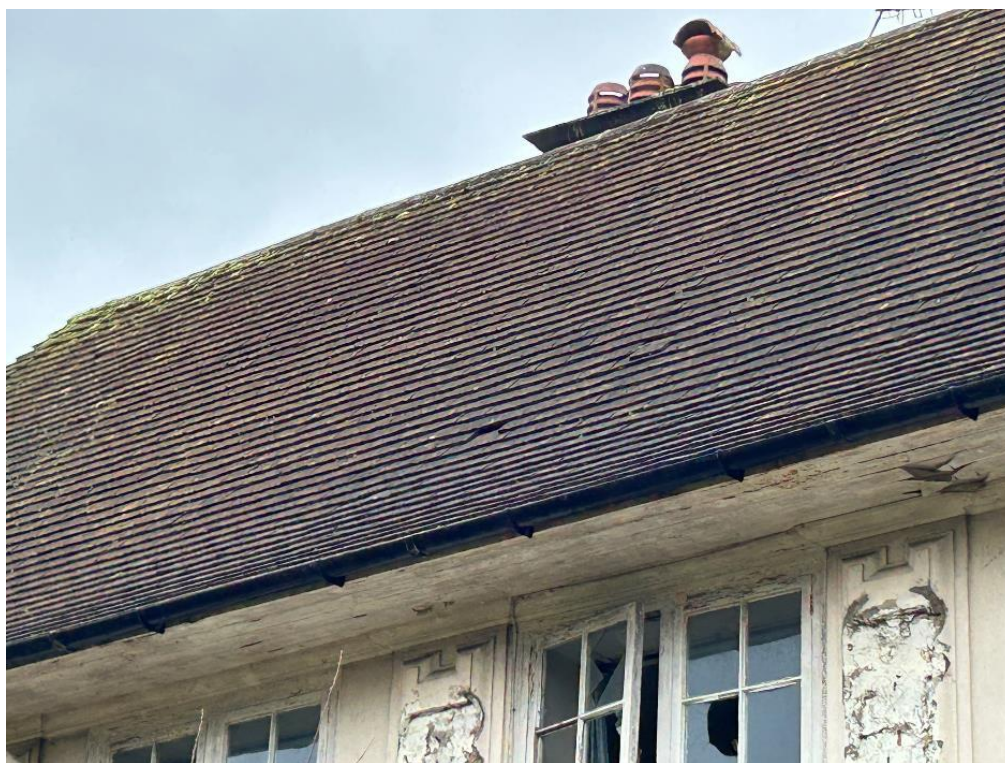
Photograph 23. B1, Missing tile
