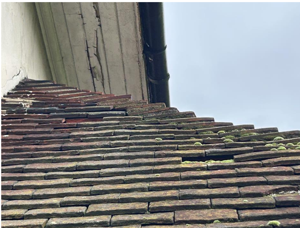
Photograph 27. B1 single-storey extension, broken tile and missing tile
