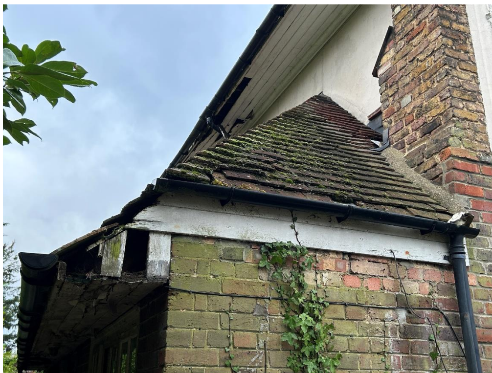
Photograph 25. B1 single-storey extension, missing tile and lifted lead flashing
