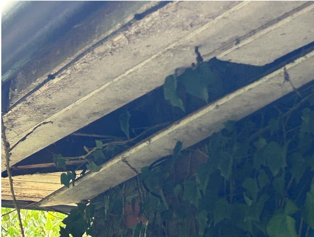
Photograph 28. Open wooden soffit of B1
