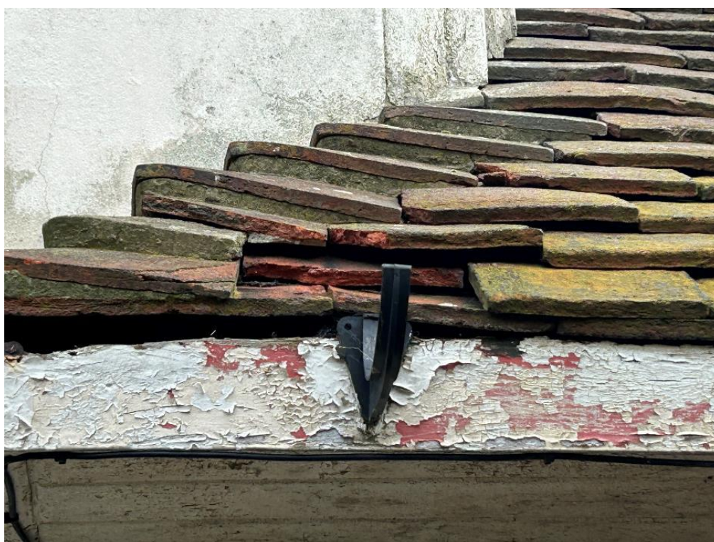
Photograph 26. B1 single-storey extension, broken tile
