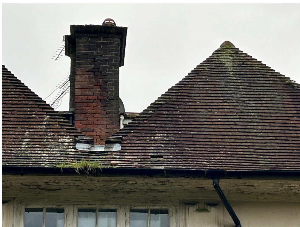
Photograph 24. B1, missing tile and lifted lead flashing
