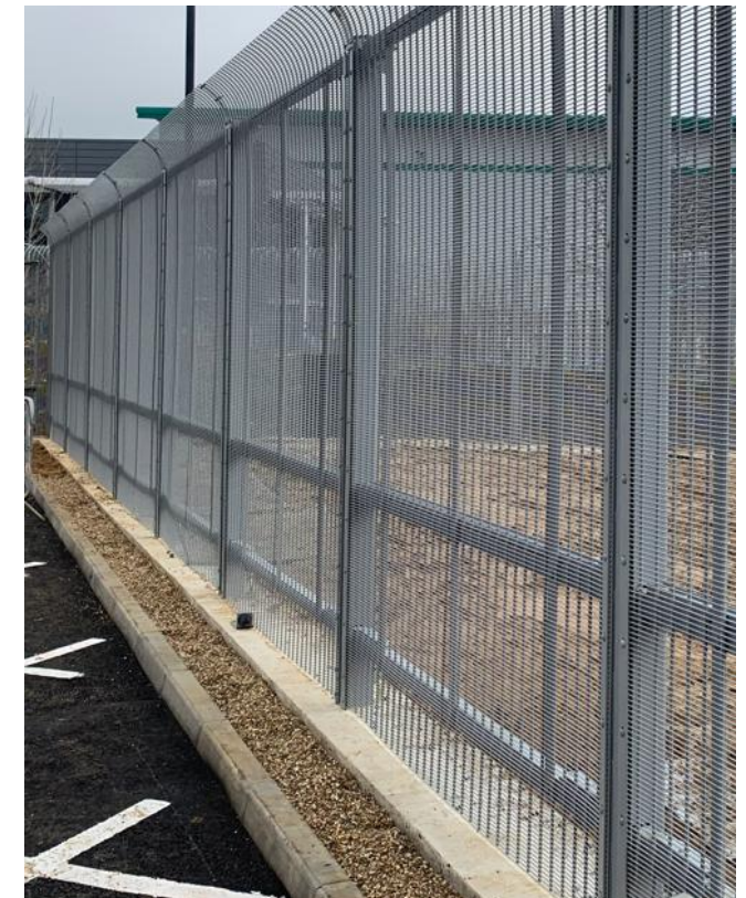
Perimeter fence – Weldmesh SecureGuard SR2 rated fence
