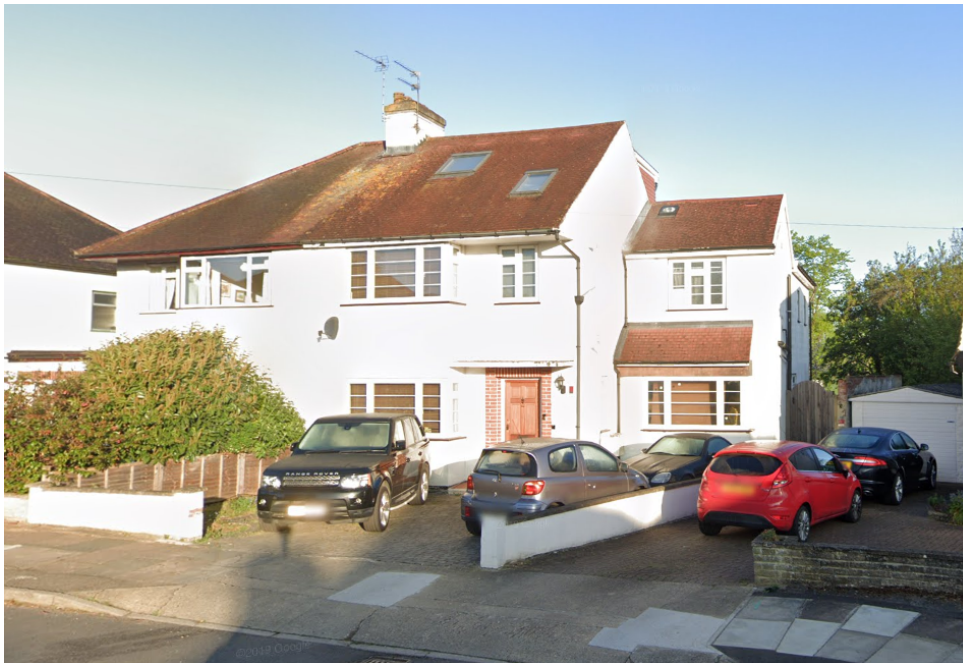
Figure 1 – Front view of existing dwelling
