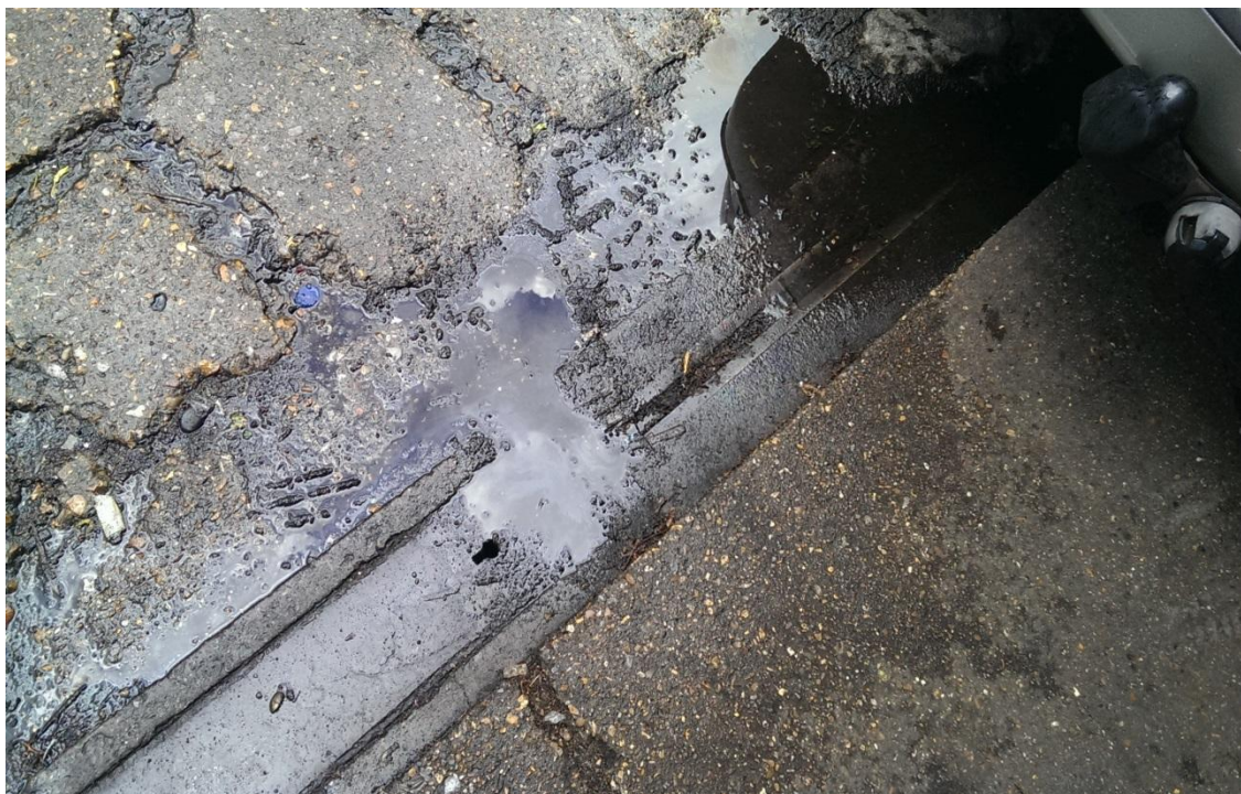
PLATE 6 – POTENTIAL HYDROCARBON SPILLAGE FROM DIESEL TANK
