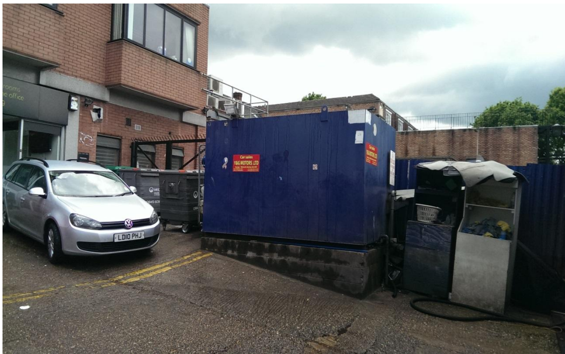
PLATE 5 – DIESEL AST ON SITE
