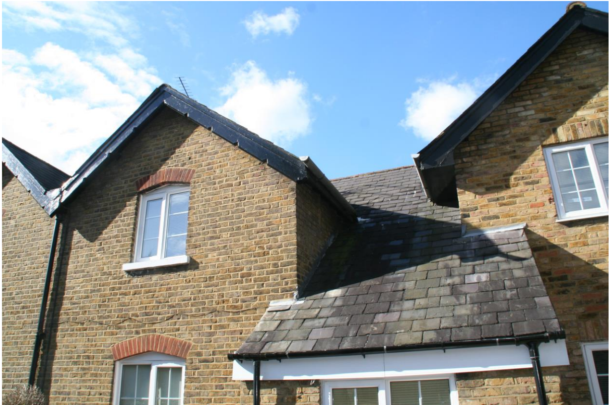
Front elevation Gabel Ends / Catslide
