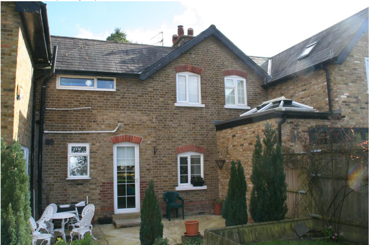
Rear Elevation (Courtyard)
