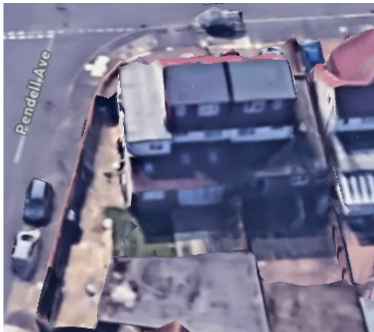
REAR AERIAL VIEW
