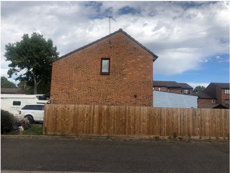
Side elevation photograph - existing (blue) timber conservatory to be demolished and replaced by proposed extension of the same depth of 3 metres
