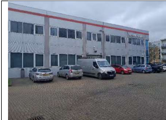
Photo 7: B1 exterior (south face).
