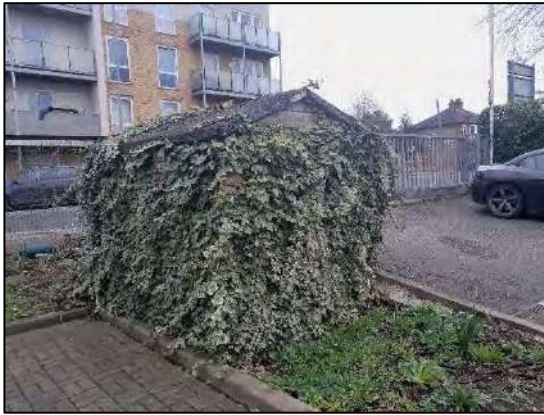
Photo 3. External view of B2
