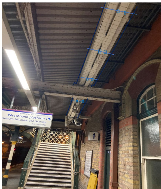
Image 13– New OPO/OTC CRMS plat 2 towards footbridge (Tailwall)
