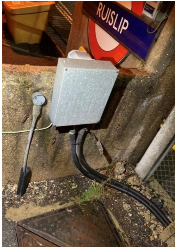
Platform 2 head wall – End State – IS Box Installed
