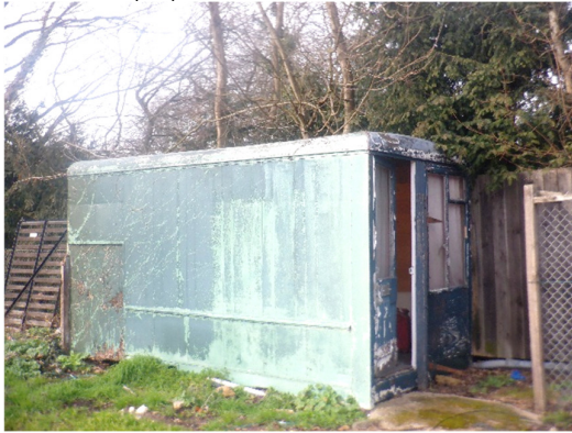
Photograph 12. Outbuilding viewed from the south (B4).
