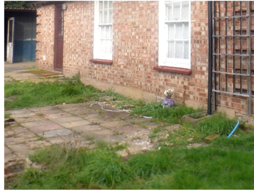
Photograph 8. Paved area on the western side of the bungalow (u1 829).
