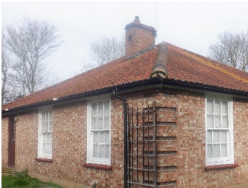
Photograph 15. Intact interlocking roof tiles (B1 - western elevation).
