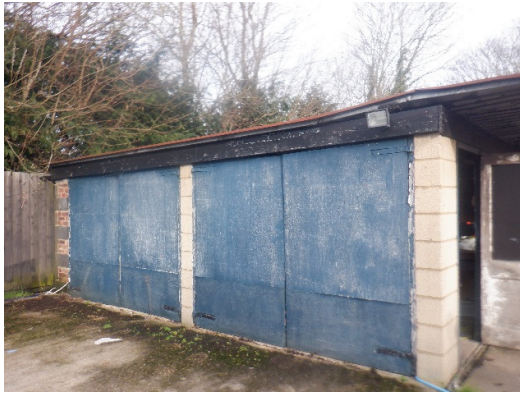
Photograph 10. Double garage viewed from the south-west (B2).
