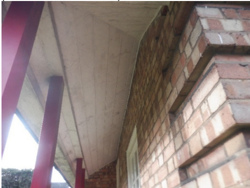
Photograph 20. Intact timber panelling of open porch (B1 – southern elevation).
