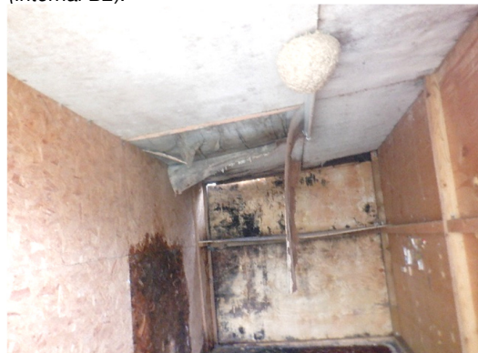
Photograph 28. Unlined roof and internal woodchip boards of B6.
