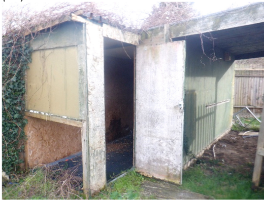
Photograph 14. Outbuilding within garden; viewed from the north (B6).
