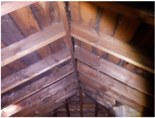
Photograph 21. Cut and pitch construction and heavily cobwebbed ridge (B1 - Roof void).
