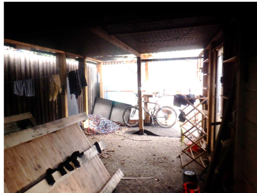
Photograph 26. Open wall at the eastern end (internal B2).
