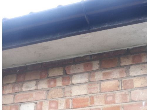
Photograph 19. Intact/tight timber soffits across the bungalow (B1 - eastern elevation).
