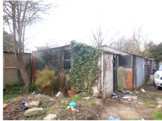
Photograph 11. Storage outbuilding viewed from the south (B3).
