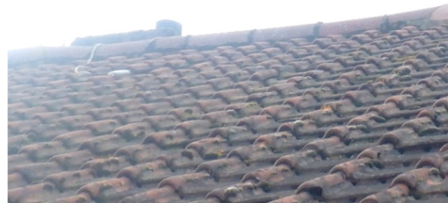
Photograph 16. Ridge mortar intact (B1 - northern elevation).
