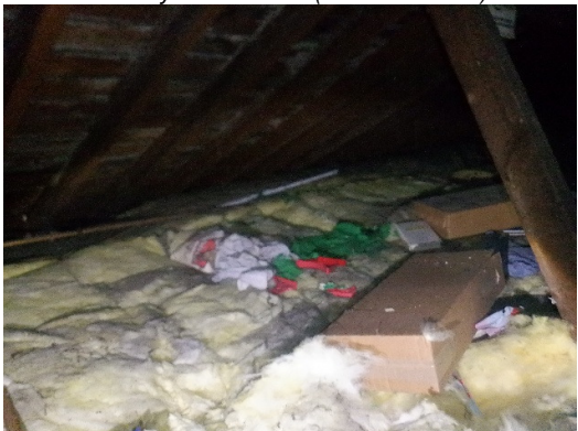
Photograph 25. Thick fibreglass between the timber joists (B1 - Roof void).
