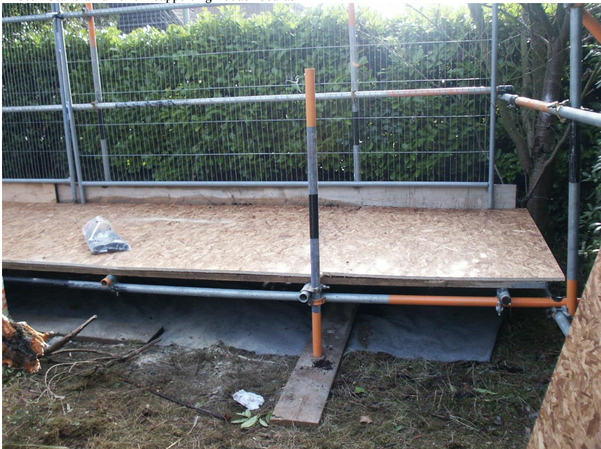
Photo 2 Scaffold framework supporting wooden boards
