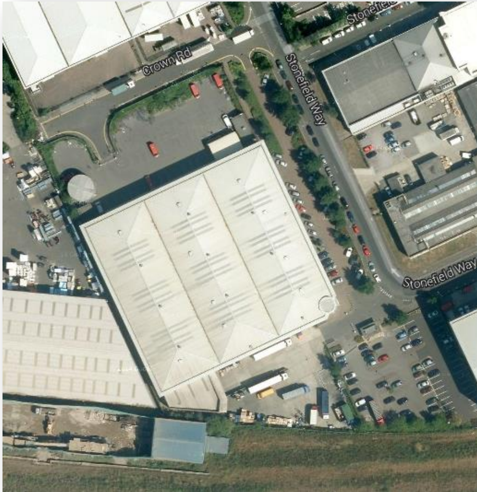
Aerial Photograph of Actual Site
