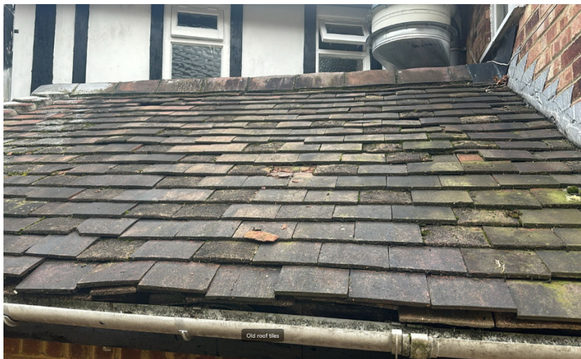
Fig 4: Existing roof tiles
