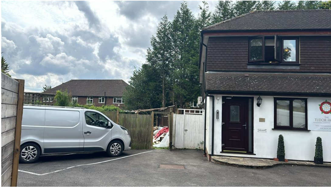
Building 3 & area of proposed development (left)
