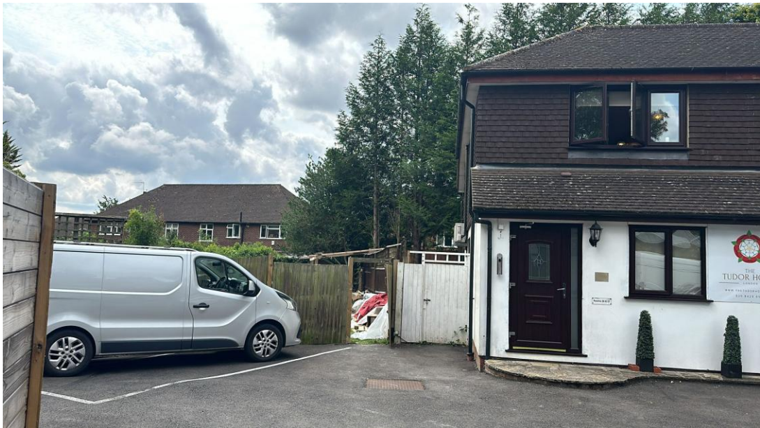
Building 3 & area of proposed development (left)
