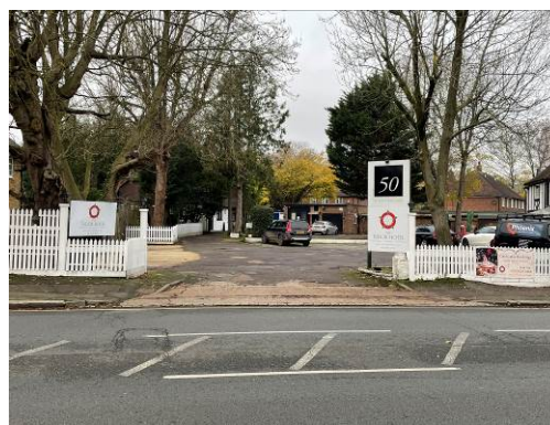
Photo 2.4 Existing site entrance
