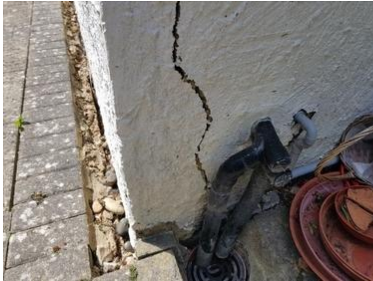
FIGURE 04 Extension left hand elevation rear corner
