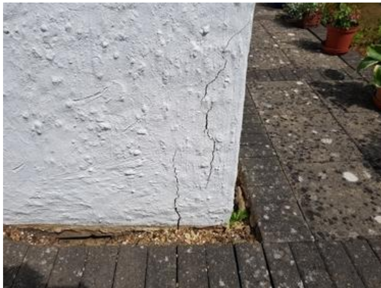
FIGURE 03 Extension right hand elevation rear corner
