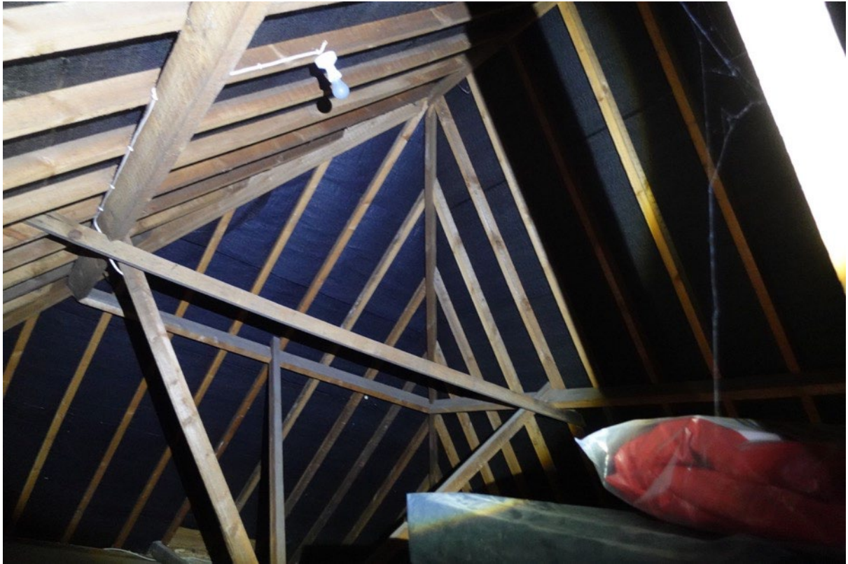
Plate 10: Black Membrane Fabric, Wooden Beams and Remains of Personal Items
