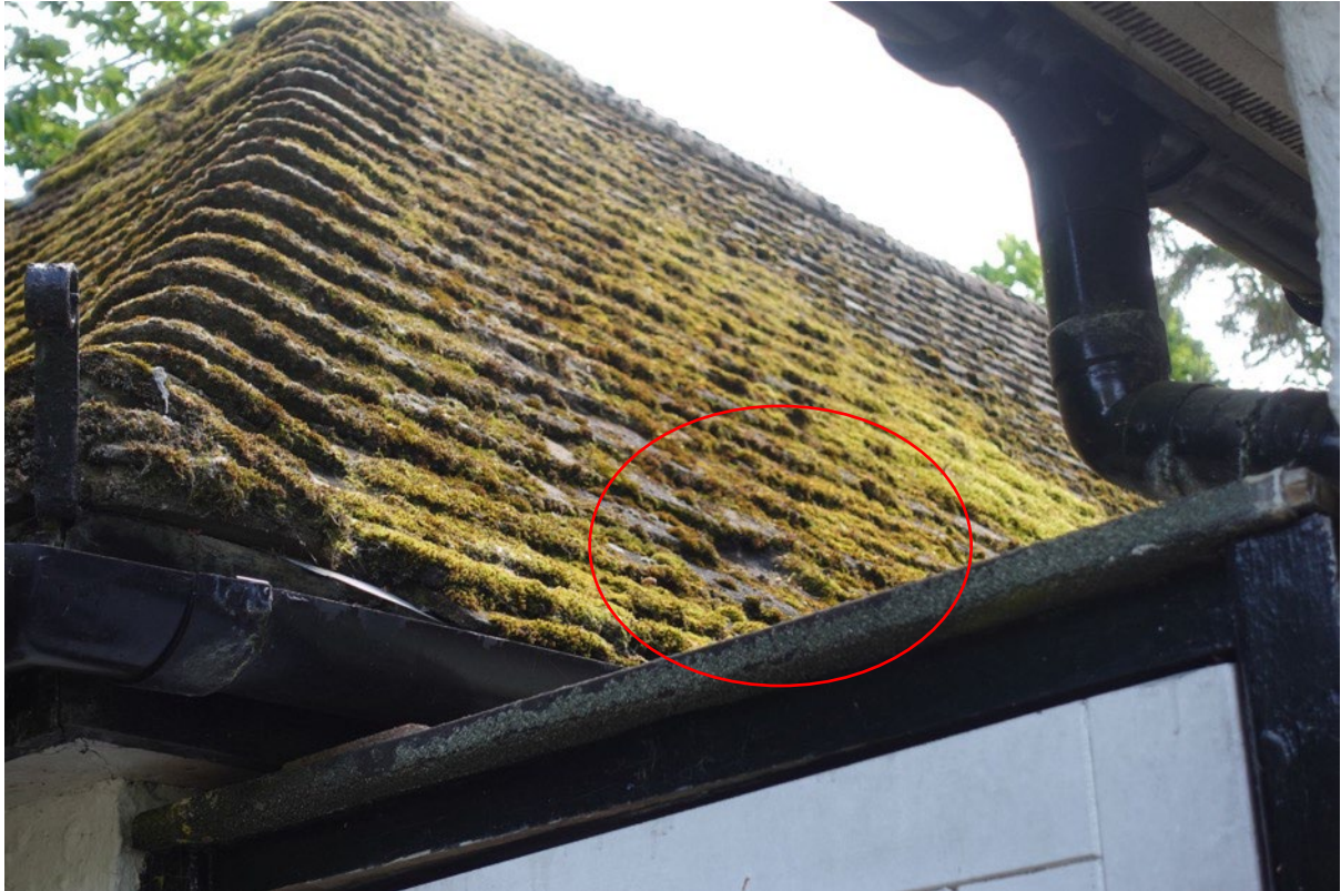
Plate 12: Missing Tile on the Garage - Western Elevation
