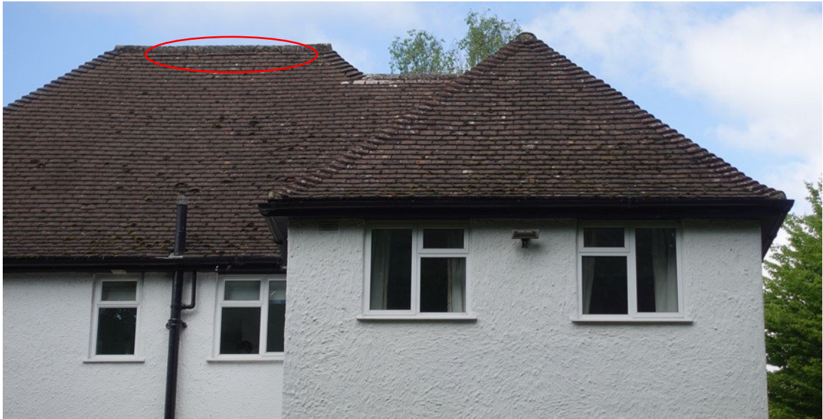
Plate 7: Eastern Elevation – Gaps noted underneath the ridge roof tiles
