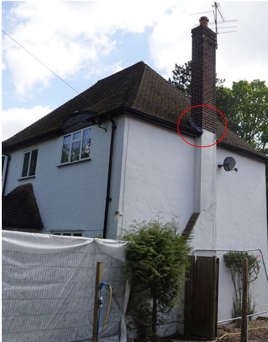
Plate 8: Southern Elevation – Lifted Lead Flashing Around Chimney
