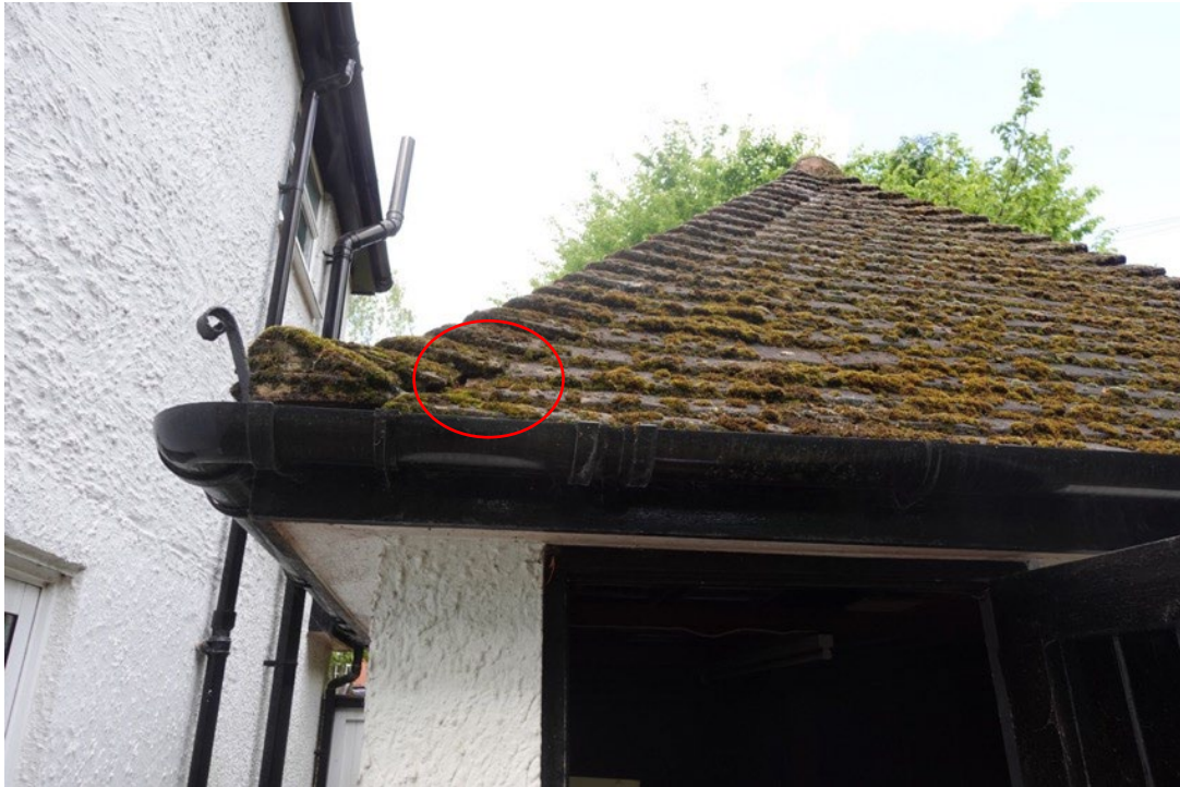
Plate 13: Missing Tile on the Garage - Southern Elevation
