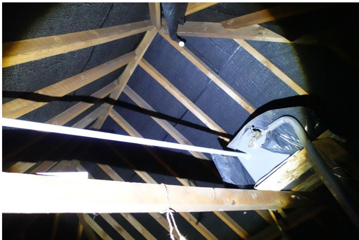
Plate 9: Black Membrane Fabric, Wooden Beams and Water Tank inside the Loft
