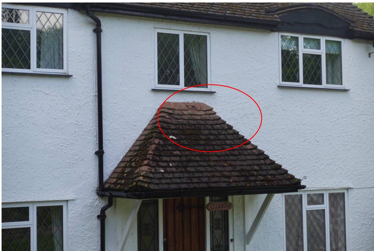
Plate 6: Broken Roof tiles on the Front Porch Roof
