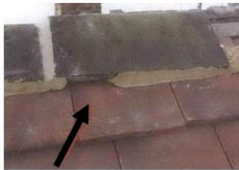
Bat Access Via Gap in Ridge Tile
