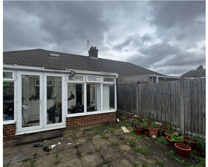
Figure 3: View towards 56 Bedford Ave from Rear Garden
