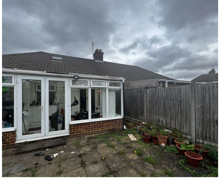
Figure 3: View towards 56 Bedford Ave from Rear Garden
