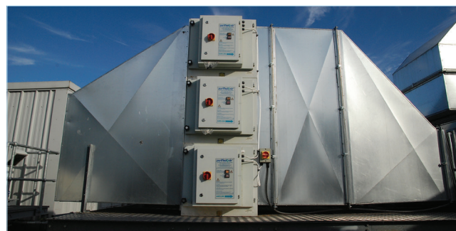
3 ESP Units Stacked in modular formation
