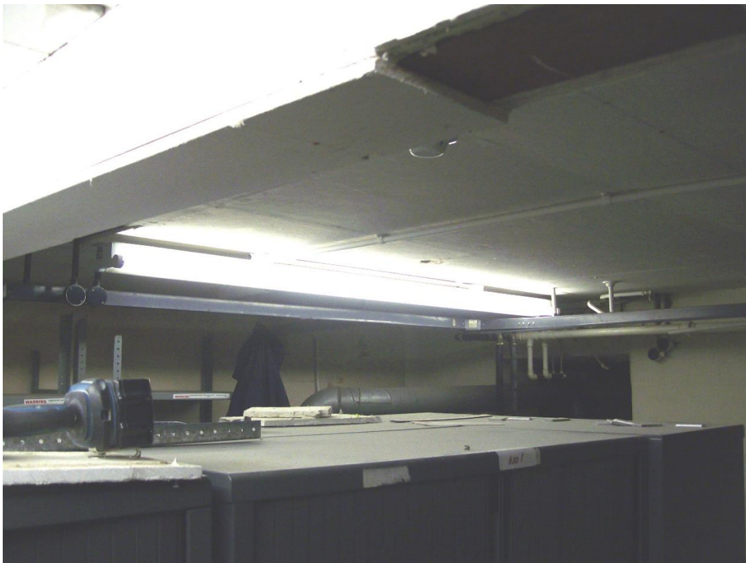
Plate 2: View of downstand steel beam providing support to timber joists at ground floor.
