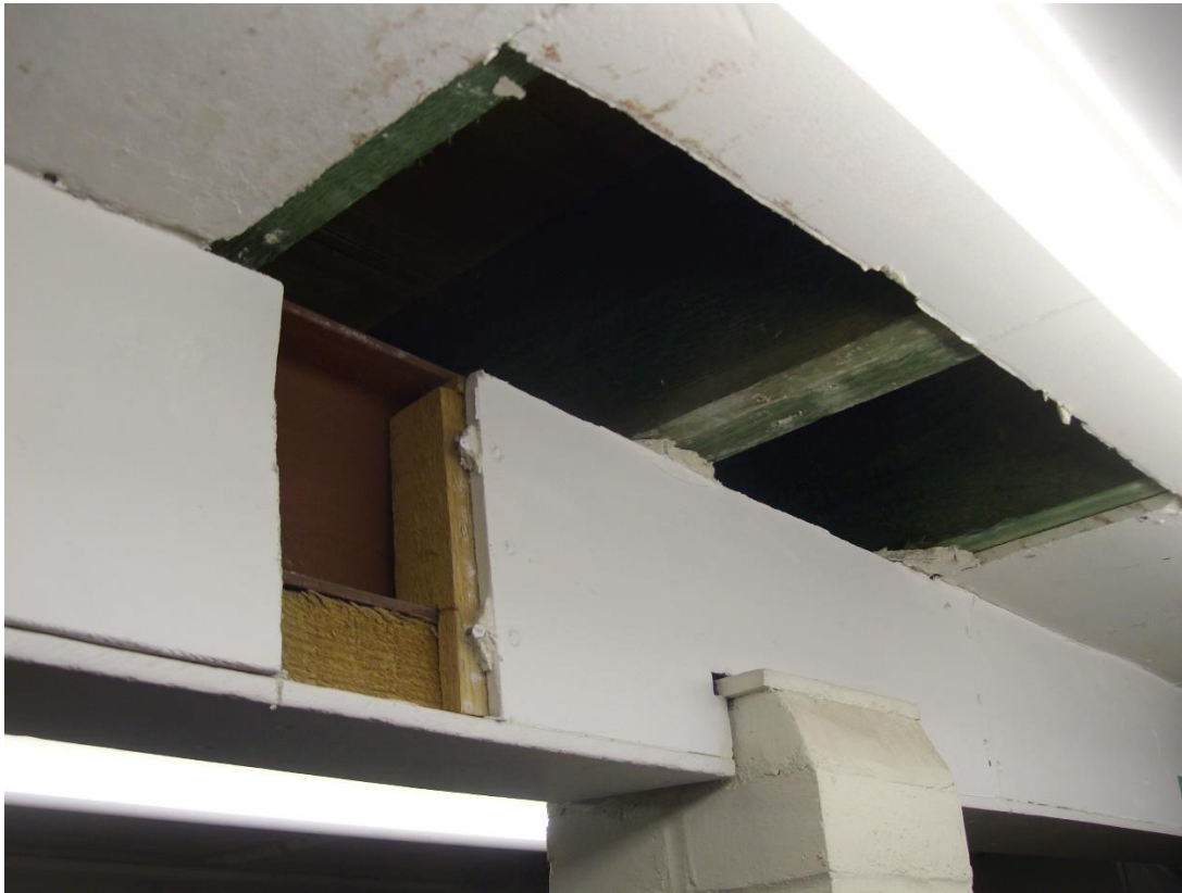
Plate 1: View of existing joists and downstand beam with local mid pier support.
