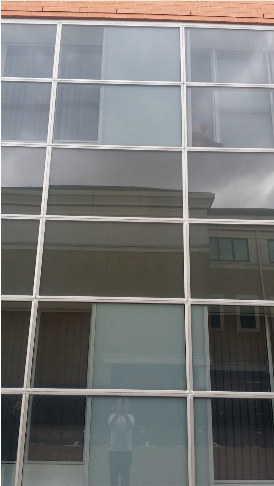
As existing - curtain walling with all 'fixed lights'
