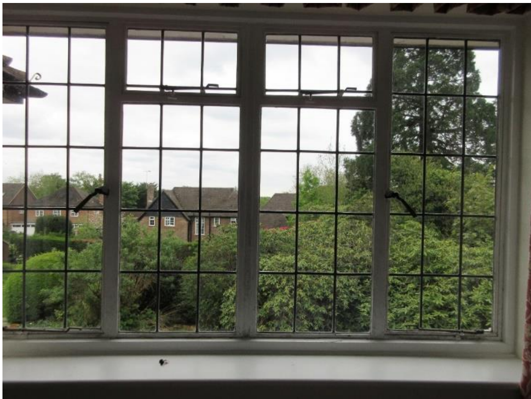
Figure 56: First floor – Metal-framed window to bedroom on west side (rear). (April 2022.)
