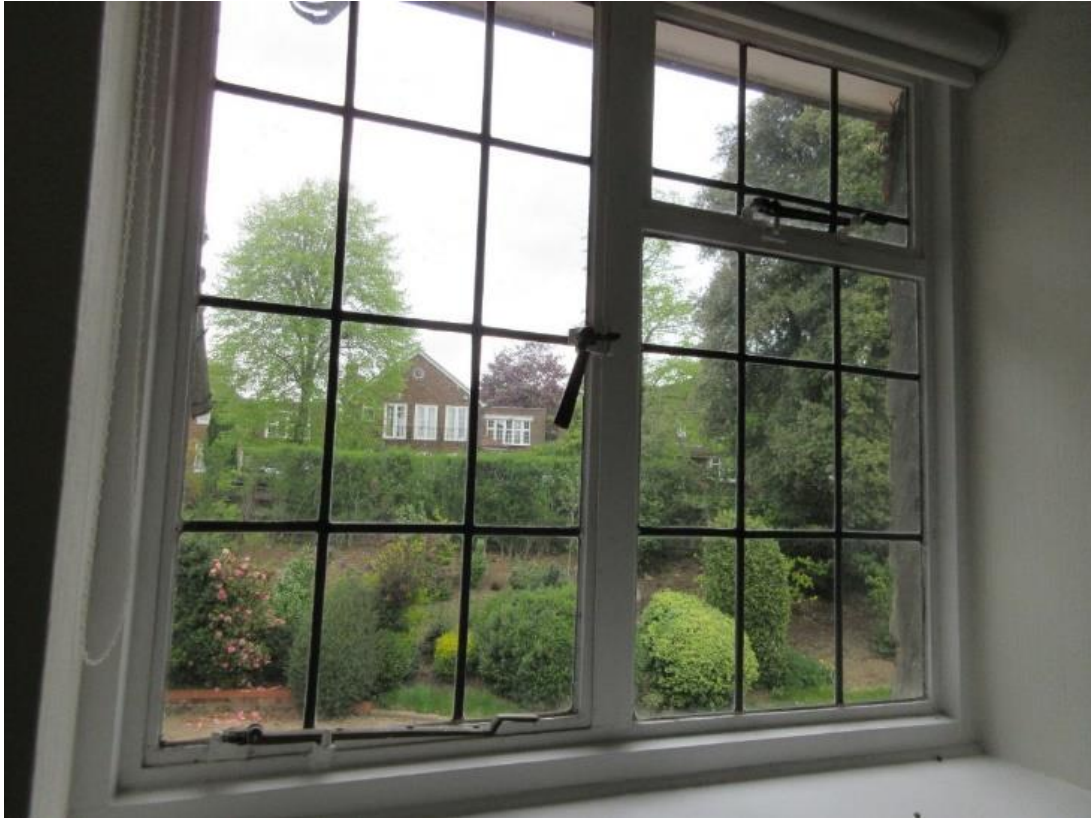
Figure 55: First floor – One of metal-framed windows to landing, facing front driveway. (April 2022.)
