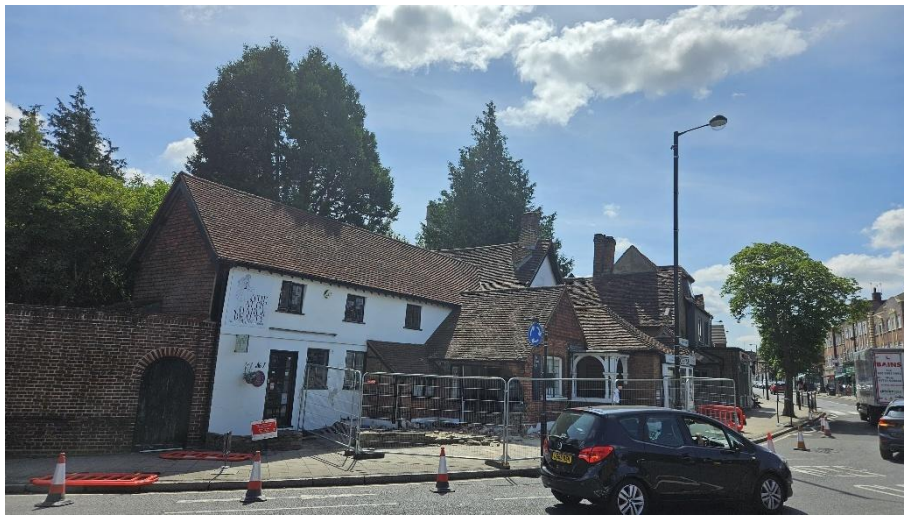
Plate 11. Overview of the damaged properties.
