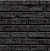
Existing black painted brick detail to remain unchanged
