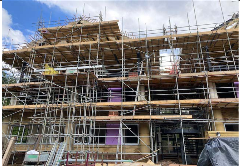
Photo 1: the building subject to redevelopment
