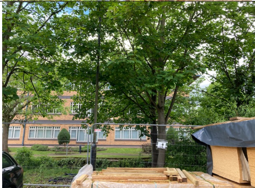
Photo 6: The mature trees along the river edge protected by tree protection fencing
