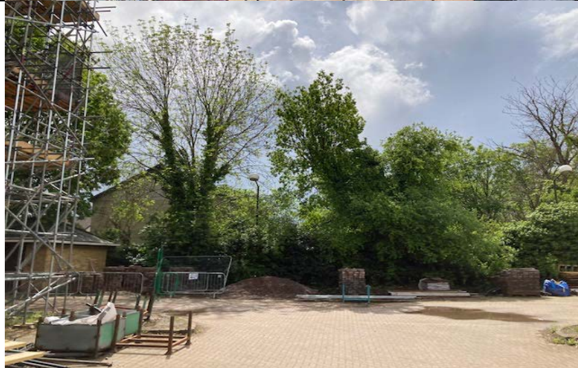
Photo 2: The southern boundary of the site, with the mature tree lines protected from the works
